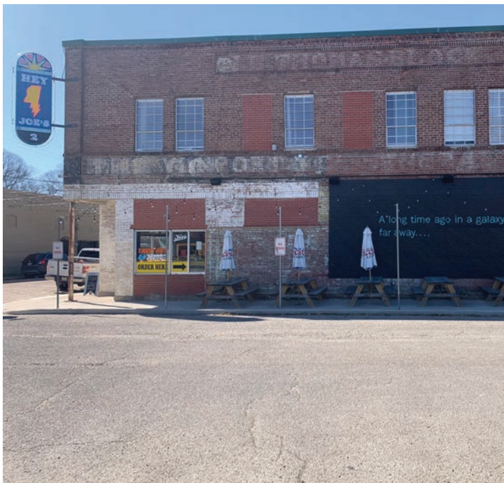
Hey Joe's in Merigold is a sister restaurant to the Hey Joe's in Cleveland. The building sits near the open field of the existing rail bed and features a mural, lighting, and outdoor seating.
