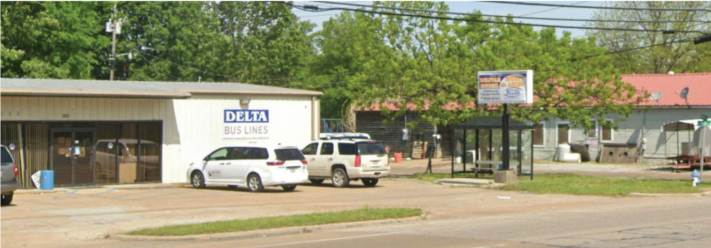
The only bus stop shelter in the three communities of Mound Bayou, Merigold, and Cleveland, is found in Cleveland. The other communities receive bus pick-ups but do not have a shelter at their pick-up locations.
