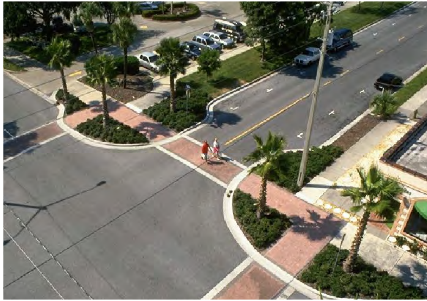
Corner bumpouts signal entry into a slower, more residential stretch of road. Creating a narrower opening onto a street signals that it is less welcoming to public use and slows traffic that may use it.
