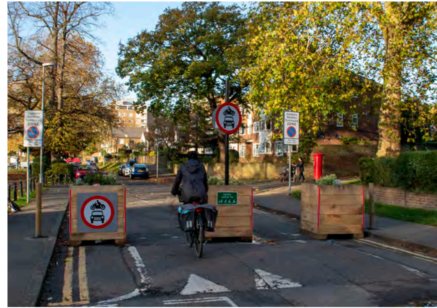
Moveable planters and bollards can be a good temporary solution as the neighborhood tests different pedestrian gateway locations. These smaller interventions are also appropriate as permanent solutions on less-frequented streets.
