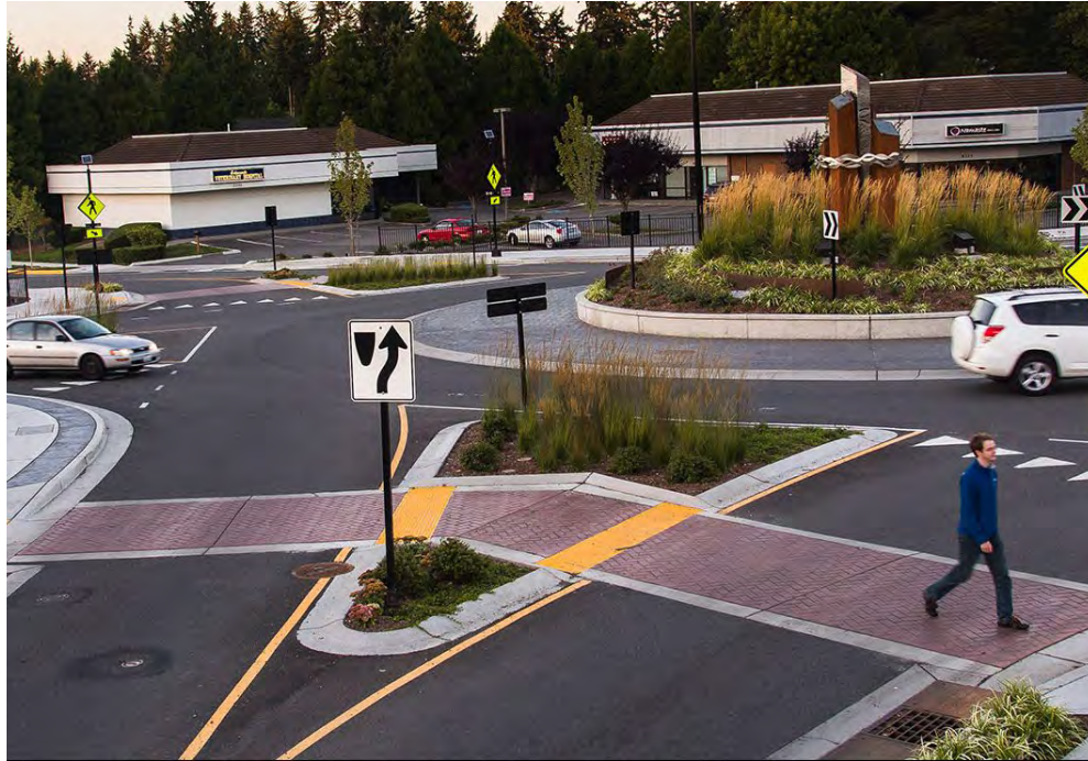
Traffic circles - or roundabouts - are extremely effective at smoothing the flow of cars. This can ease traffic buildup at these busy intersections, taking the pressure of traffic backup off of connecting streets.
