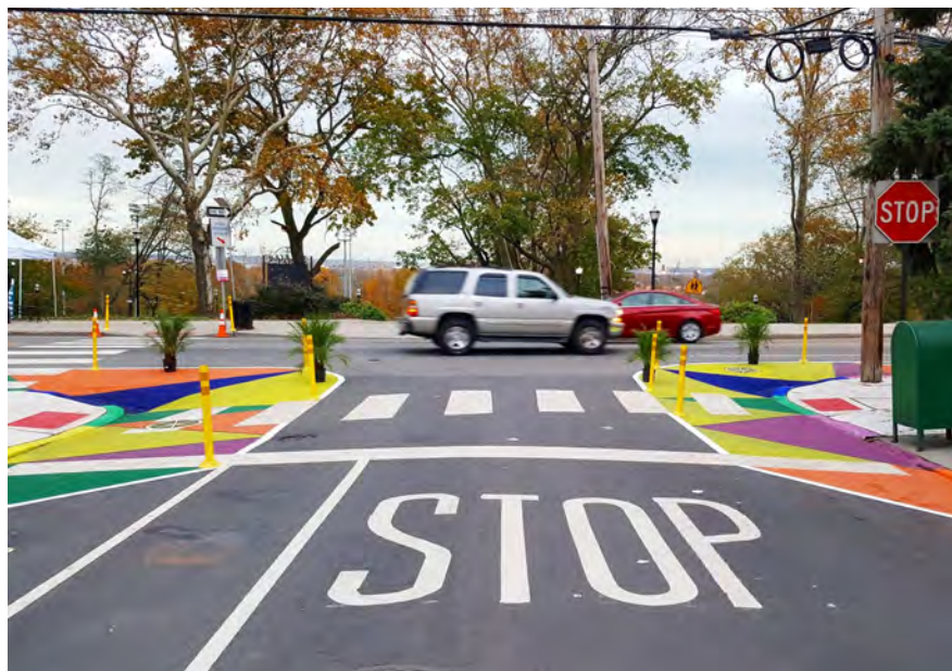
Where it is not possible to fully construct corner bumpouts, painted bumpouts with bollards, planters, and other temporary barriers can be an effective (and colorful!) alternative.
